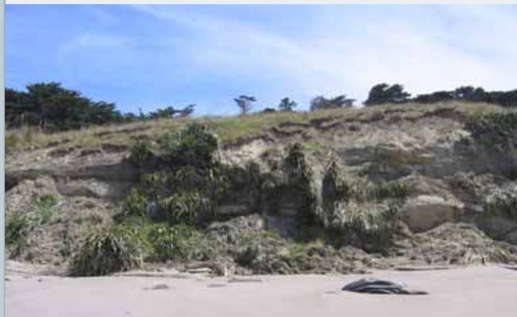
Erosion near Otahome
