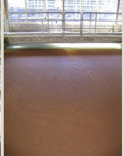
Float layer over filter
