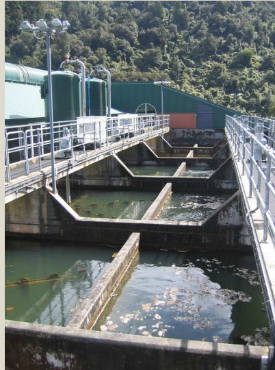
Flocculation tanks
