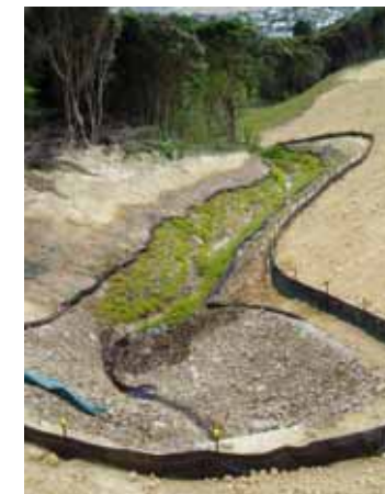
A good example of a stream diversion with sediment control, natural looking 'new' channel and planting
