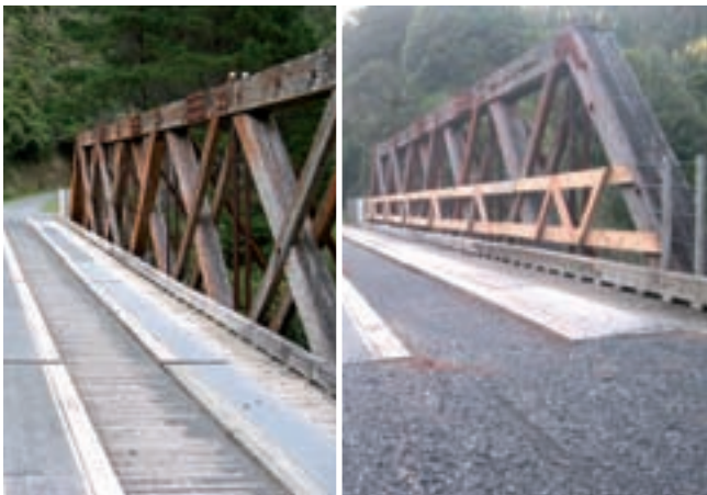
Pakuratahi Truss Bridge before handrail... and after handrail installed
