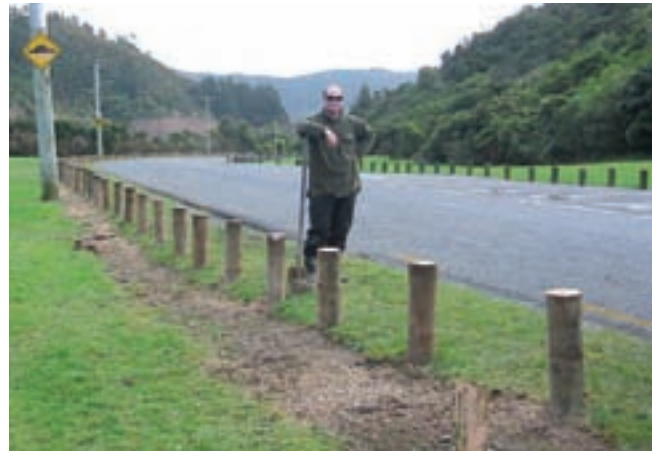
more permanent bollards were installed
