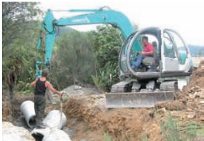
Tunnel Gully culvert pipes were upgraded
