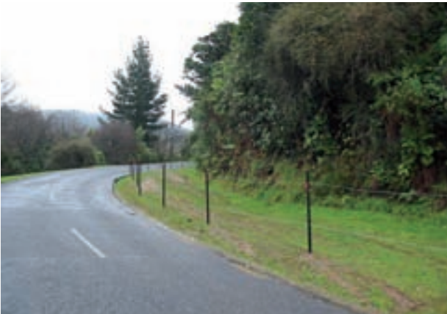
A temporary fence was put in before...
