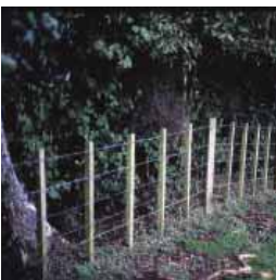
A sturdy 7 wire post and batten fence will keep most stock out of your bush block.
