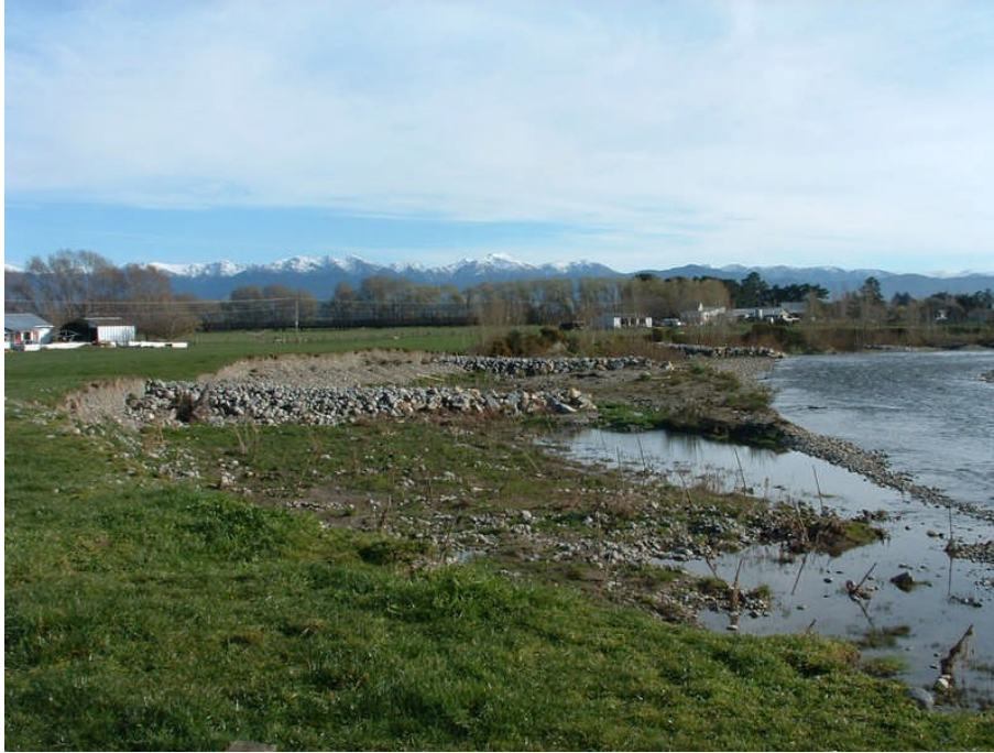
Photo 1: Boulder groynes adjacent to Daniel's property
