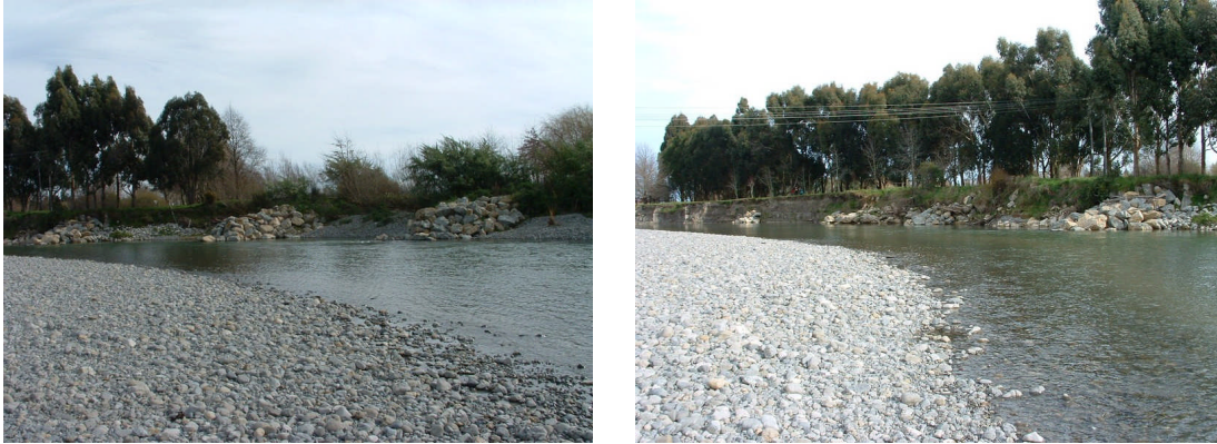
Photo 5: Looking upstream and downstream at boulder and shingle groynes.
