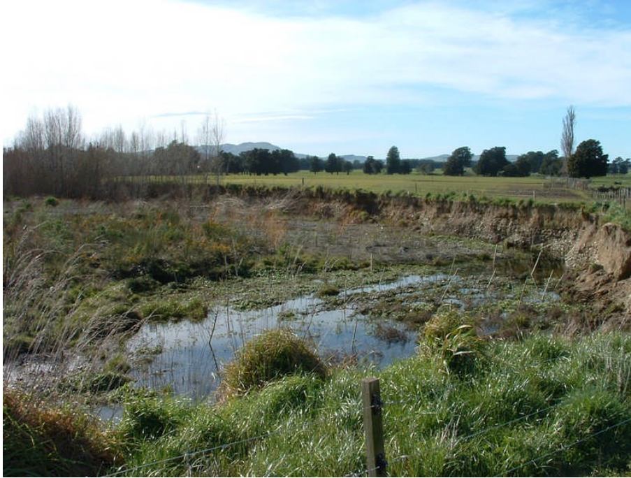
Photo 3: Lateral erosion at Buick property, newly planted willow poles.
