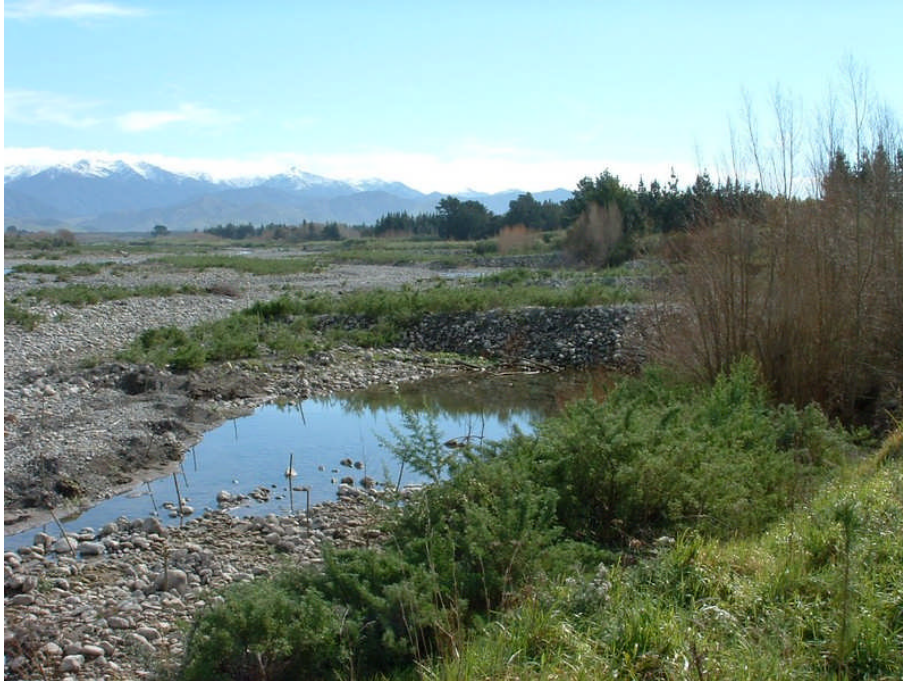
Photo 4: Shingle groynes & willow plantings.
