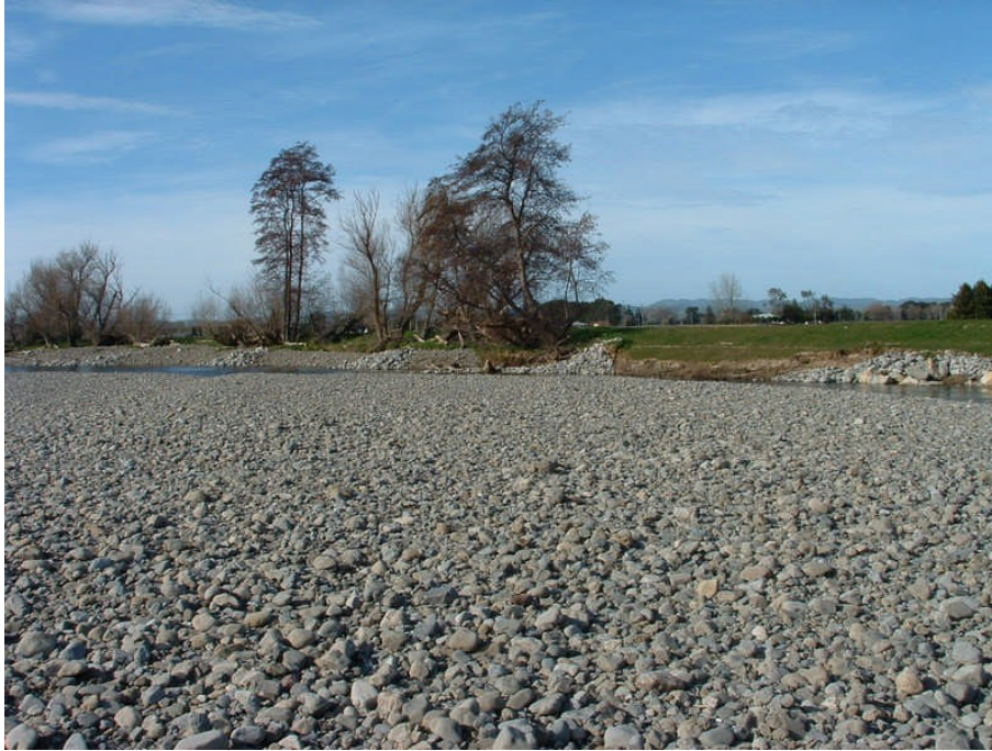
Photo 2: Boulder and gravel groynes. Note lateral bank edge erosion & large gravel beach.
