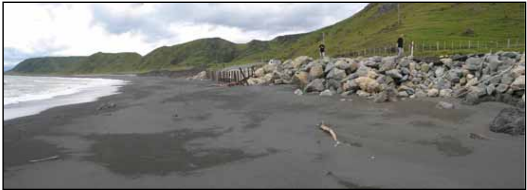
Figure 5: Existing erosion control measures to be replaced as "priority 1" works
