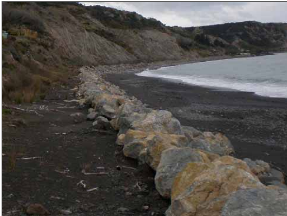
Figure 2: Existing Boulder Beach
