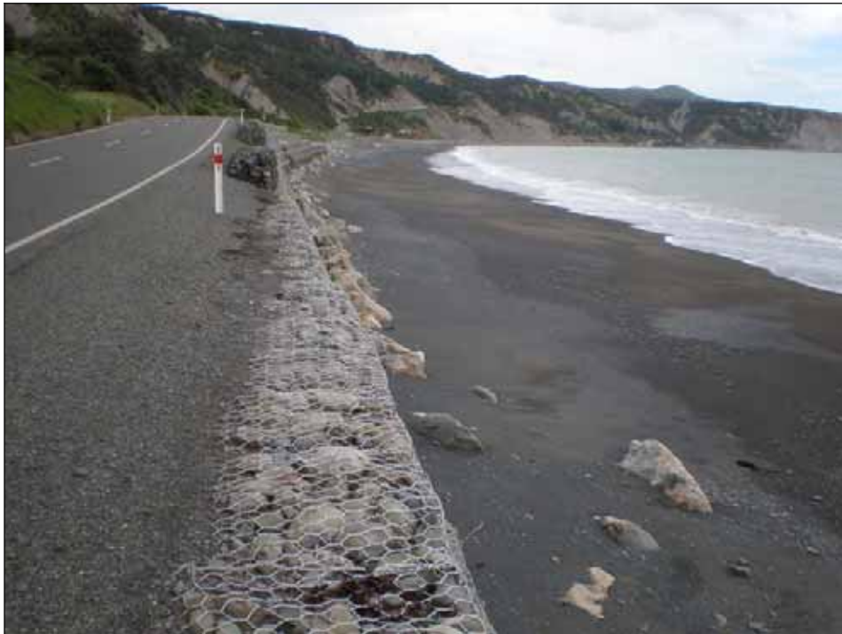
Figure 4: Existing Gabion Wall
