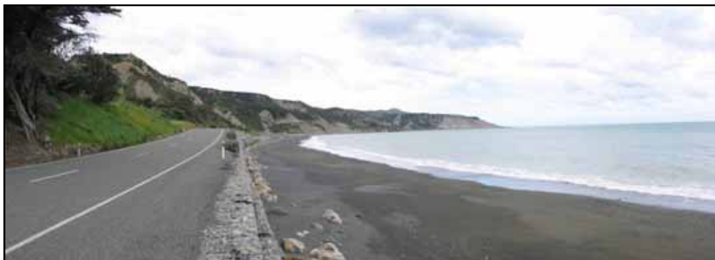
Figure 2: Existing section of sea wall (gabion baskets) south of Te Kopi
