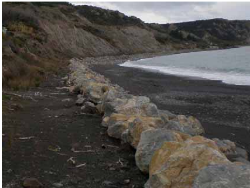
Figure 2: Photograph showing existing boulder beach material
