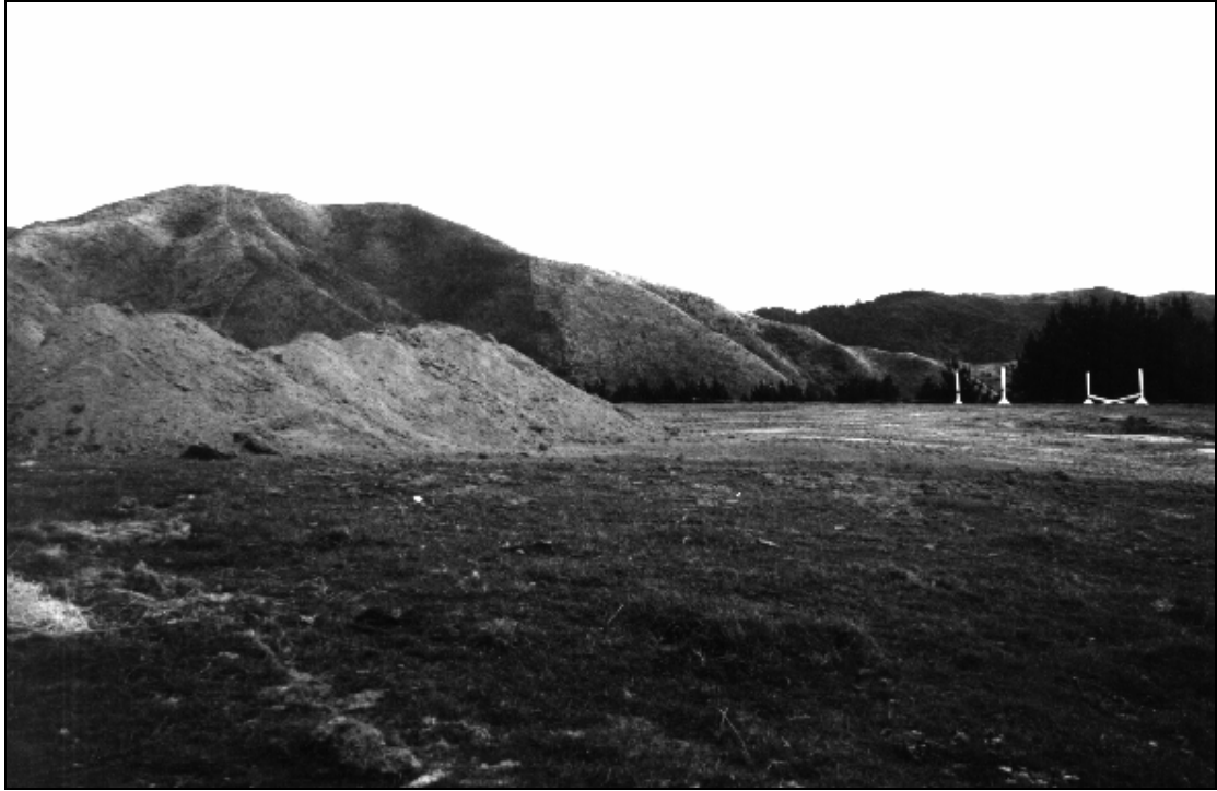
Figure 26: Unconsented Earthworks at Waikanae on 13 May 1997
