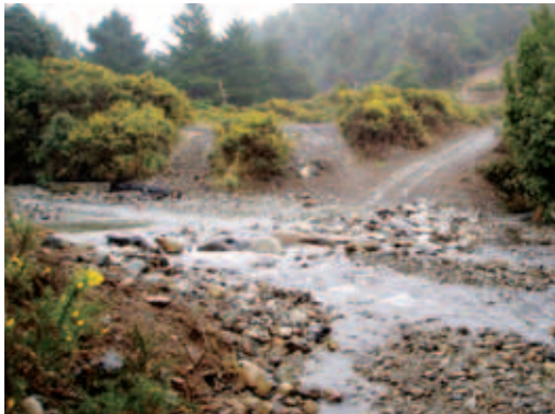
Ford after lowering – removal of barrier to fish passage
