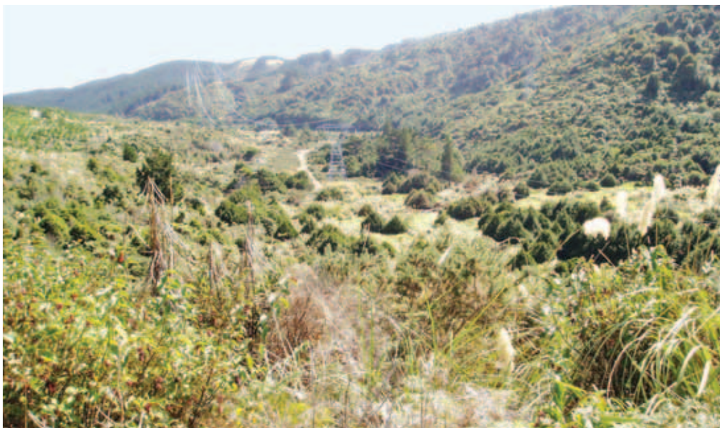
Pylons crossing Akatarawa Forest
