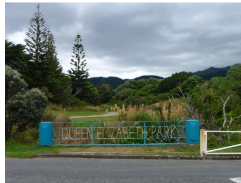
Figure 24: Bespoke Railings at Paekakariki entrance
