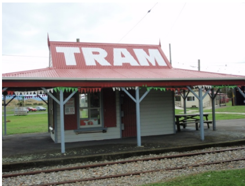
Figure 23: Existing Tram stop at Mackay Crossing
