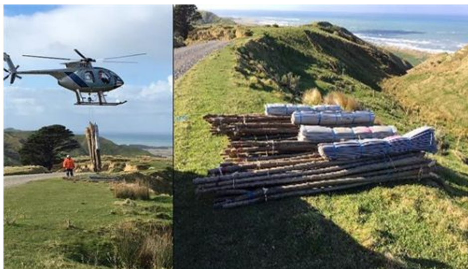
Flat Point Farm delivering poles to site
