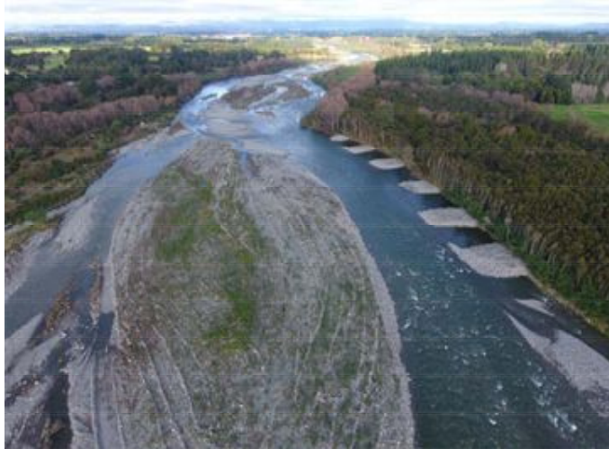
Photo 1: Waingawa gravel groynes at cross section 26
