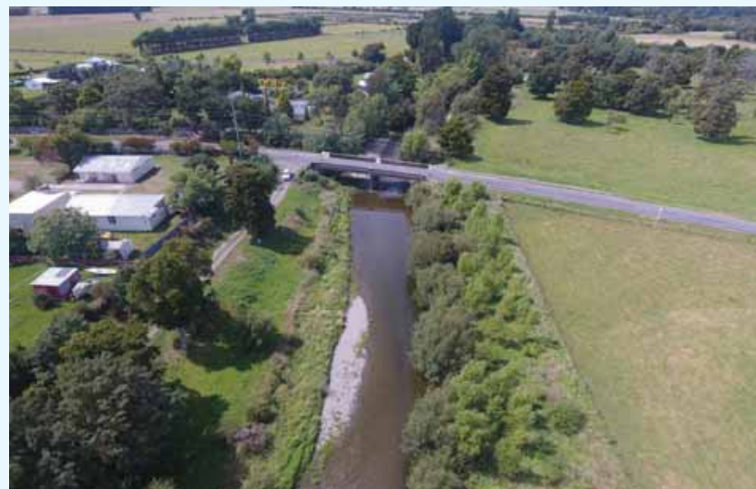
Paierau Road Bridge
