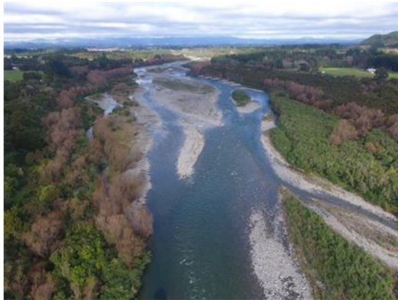
Programmed work completed in the Waingawa River Scheme
