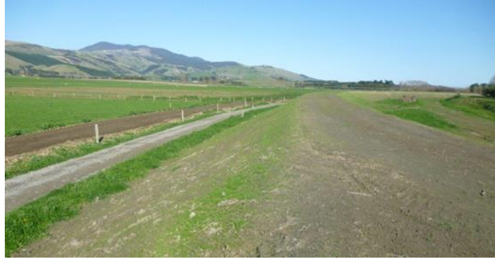
Stage 1 Construction 1 complete
