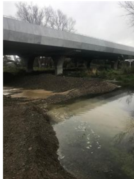
Waikanae Expressway Bridge: Diversion cut and extraction
