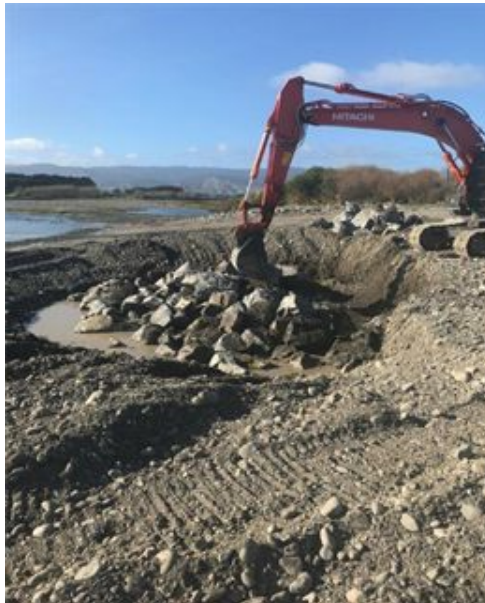
Otaki river rock groynes under construction
