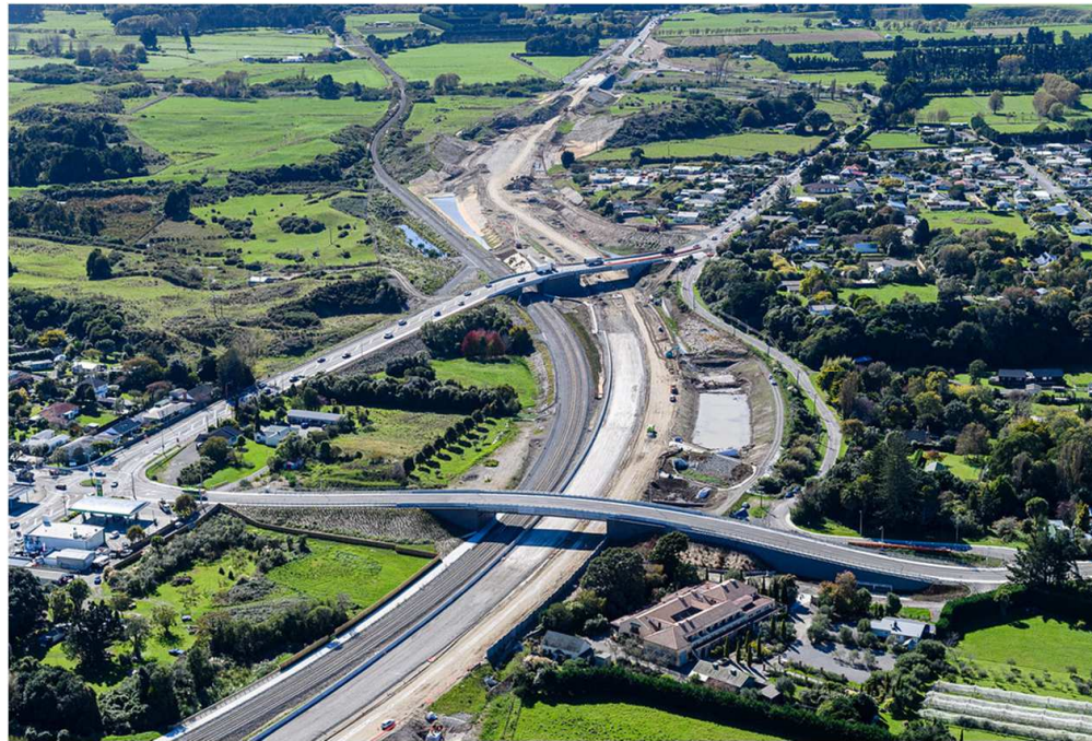
View of Rahui Road and SH1 north
