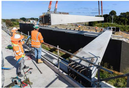
First beams being laid on Bridge 9
