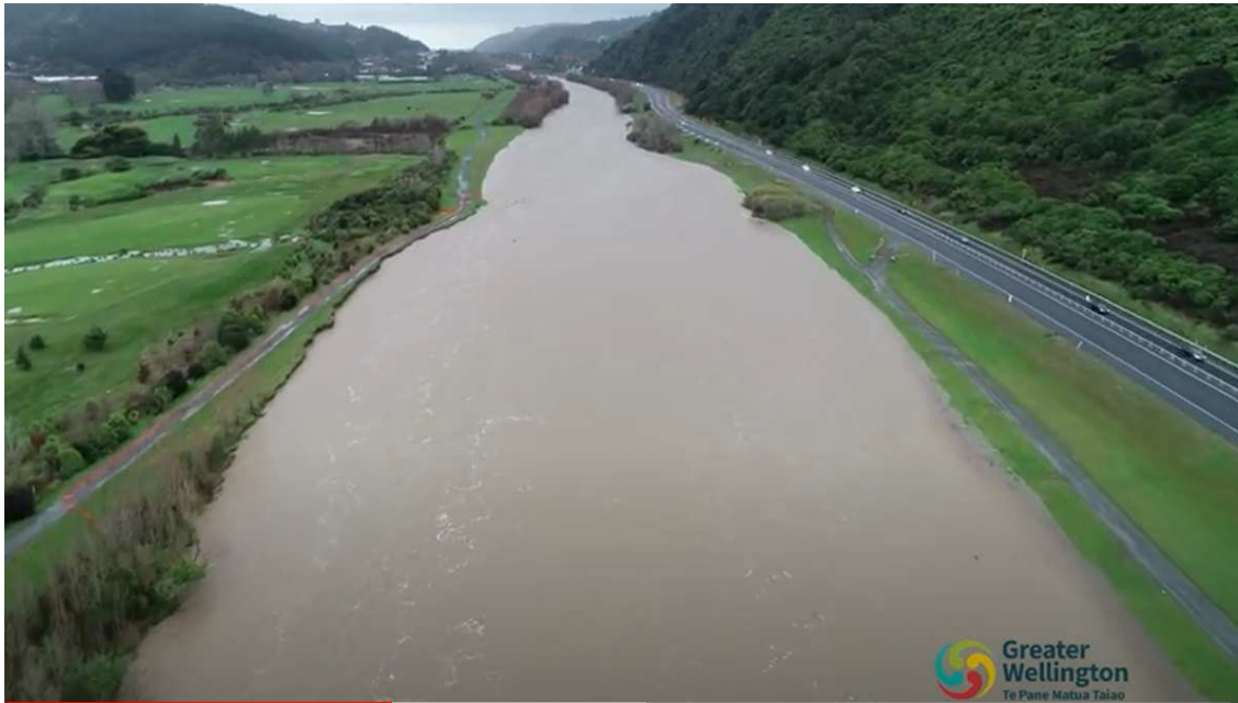
Figure 3: Erosion area adjacent to the Royal Wellington Golf Club 18/7/21 (Erosion area left of photo, view looking downriver)
