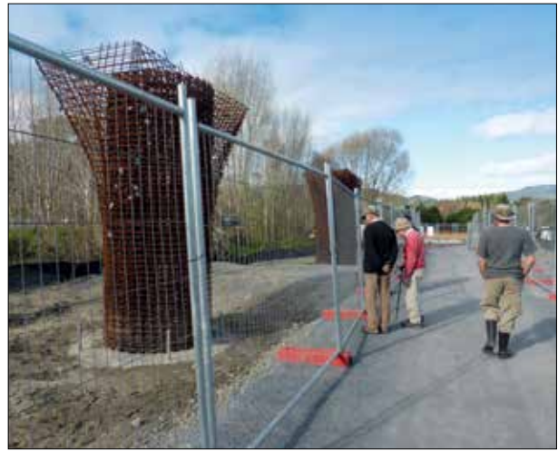
Construction of the Expressway bridge
