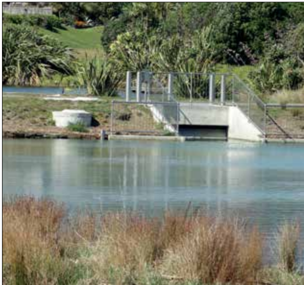
The Waimanu Lagoon floodgate now allows for fish passage
