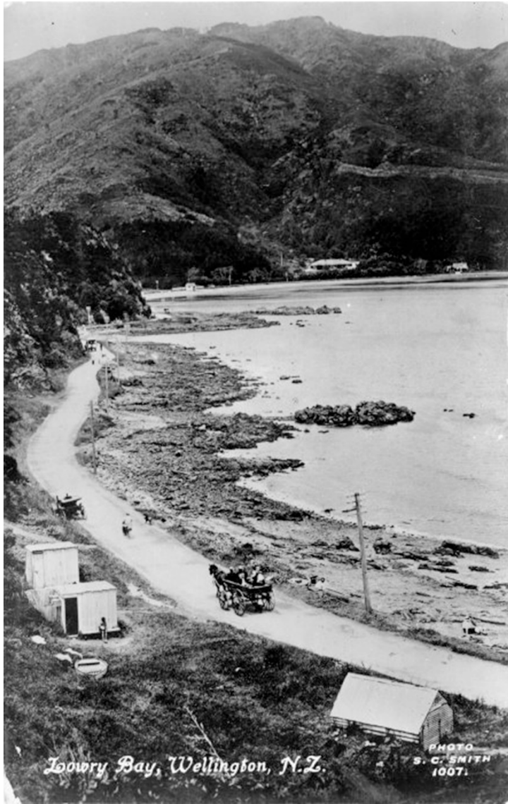
Figure 3: Lowry Bay 1920 Turnbull Library
