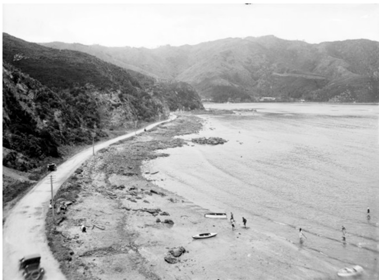
Figure 4: Lowry Bay 1920 Turnbull Library
