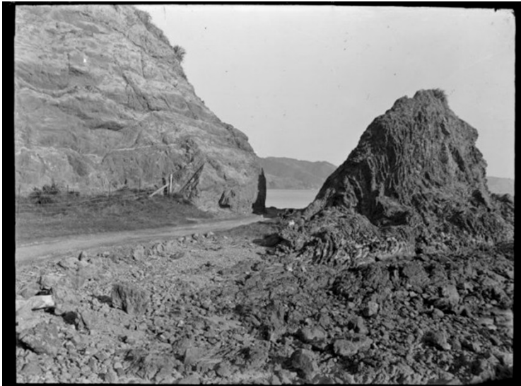
Figure 1: Lowry Bay 1905 Turnbull Library
