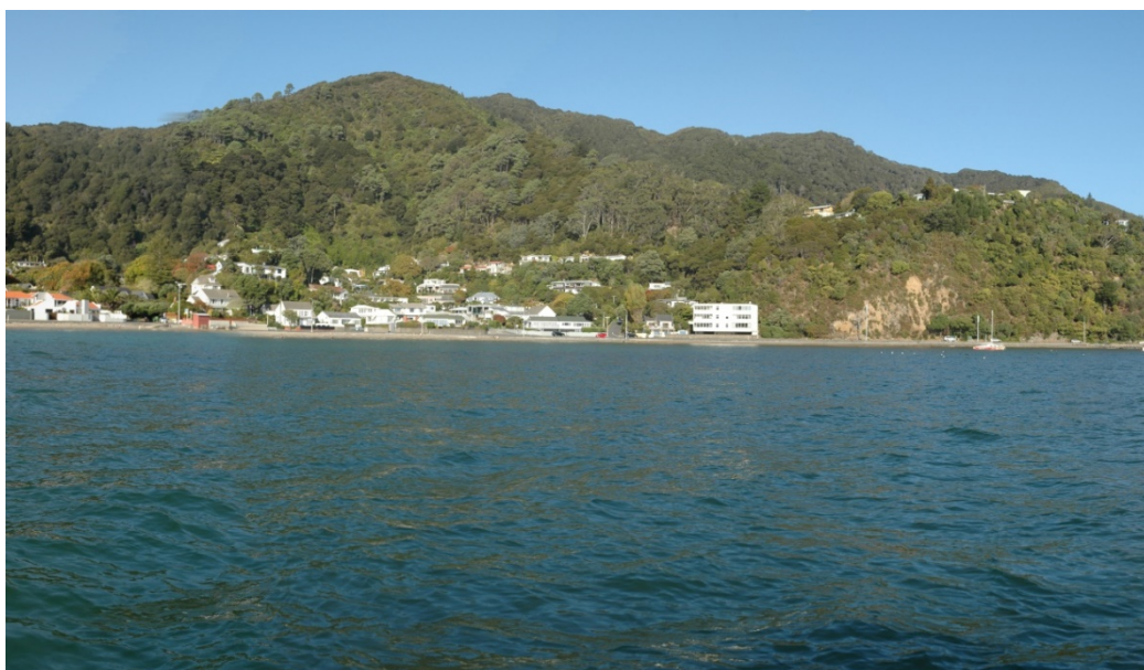
Figure 21: Taken 250m from Lowry Bay beach. The Whiorau Bay revetment is behind the boats to the right of the photograph.
