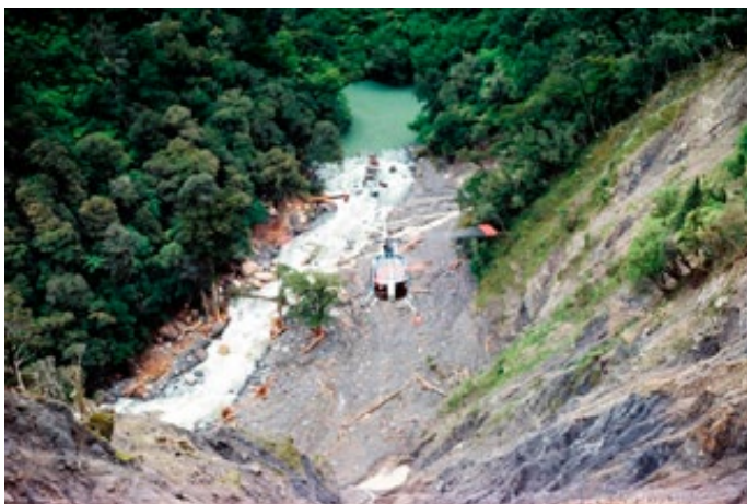
Figure 21: Landslip in gorge during 1982 flood – GWRC.
