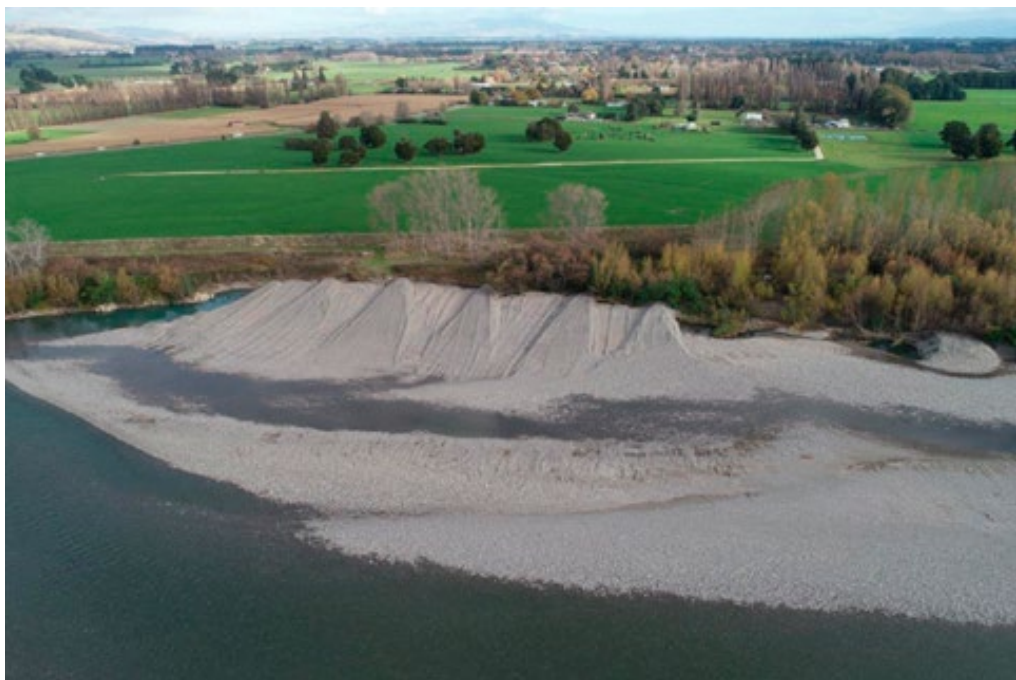
Figure 87: Critical Area Photograph – Platform Farm – GWRC.
