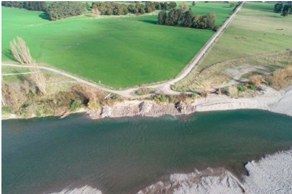
Figure 88: Critical Area Photograph – Kuratawhiti Street – GWRC.
