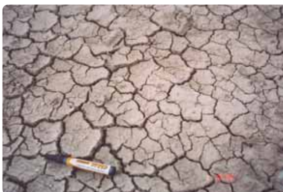
* Cracking clay soils - self regulate with wet and dry cycles
