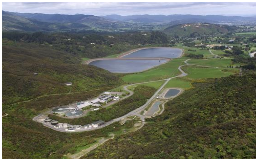
Figure 11 Te Marua treatment plant and Macaskill lakes
