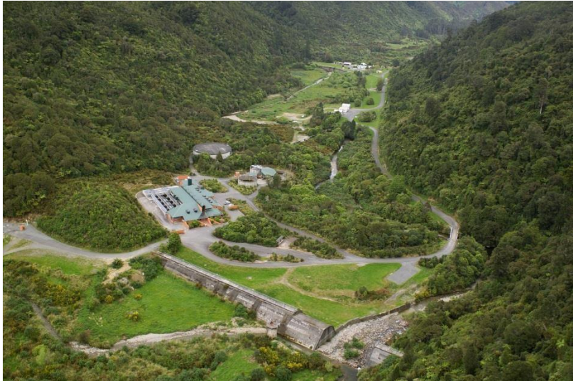
Figure 12 Wainuiomata treatment plant
