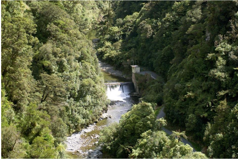
Figure 10 Kaitoke intake on the Hutt River
