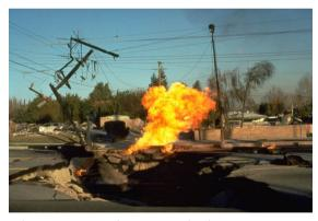
Above: A gas main ruptures in the 1994 Northridge earthquake.
