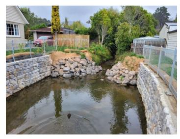
Figure 9 Redi-Rock walls and scour protection upstream of Sunbrae Culvert (photo credit: GHD)
